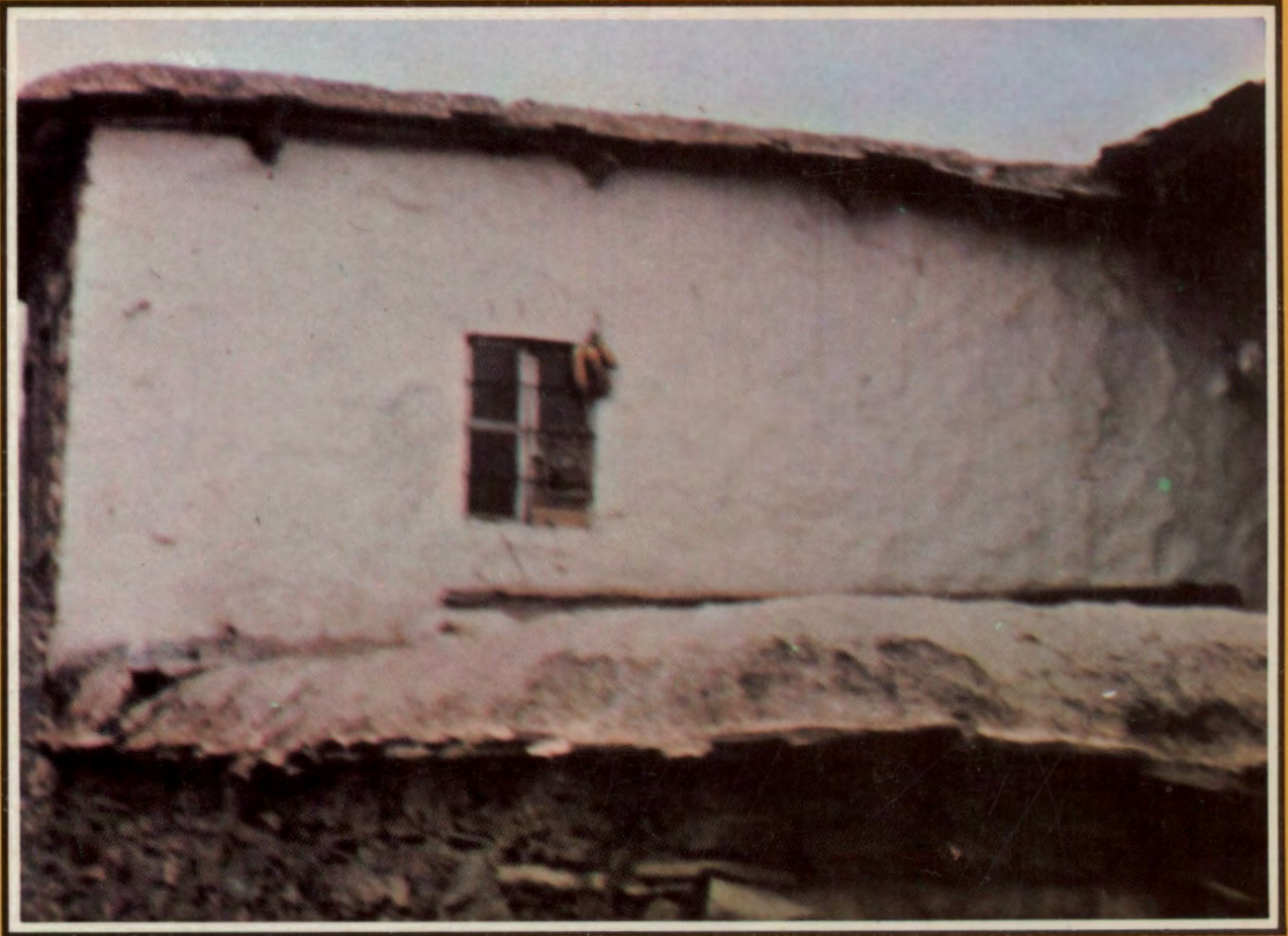
A house in a village which is plastered with asbestos mixed white soil.
