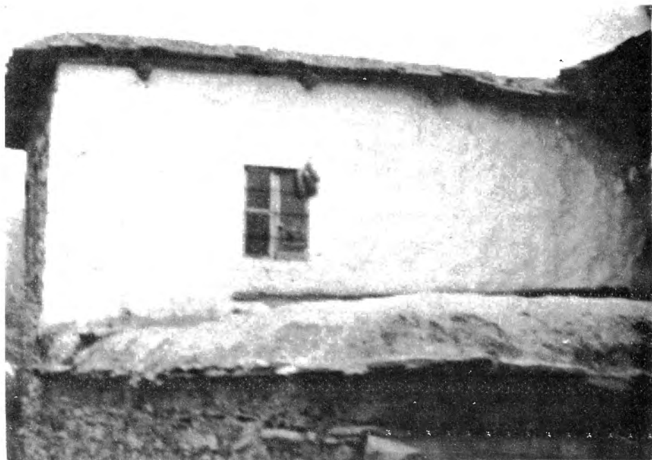
Figure 6. A house in a village which is plastered with asbestos mixed white soil.
